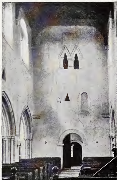
86. INTERIOR OF DEERHURST TOWER
